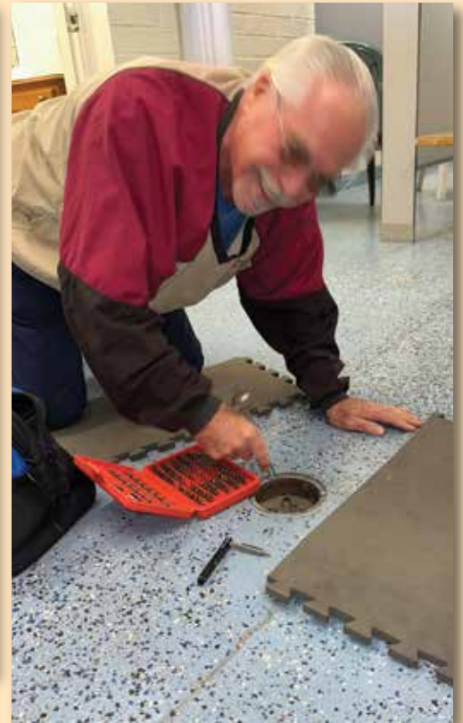
Dan Martini repairs a clean out drain cover
